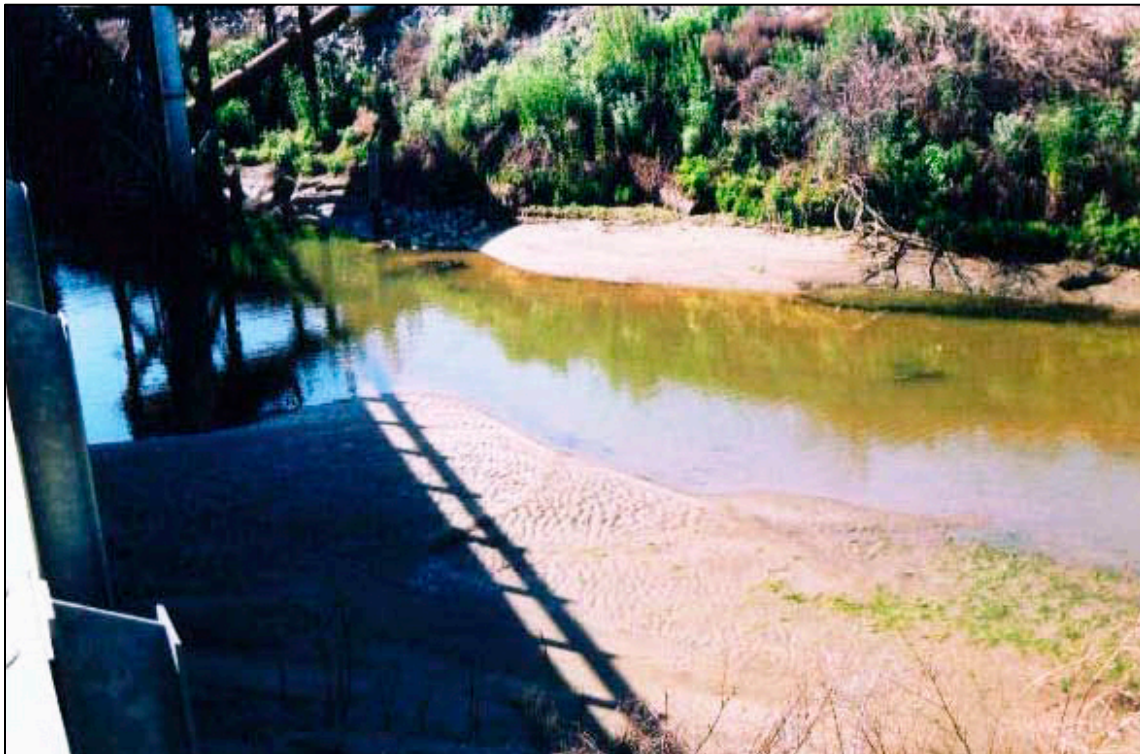
Figure 6 Middle River at Undine Bridge, April 1, 2007
